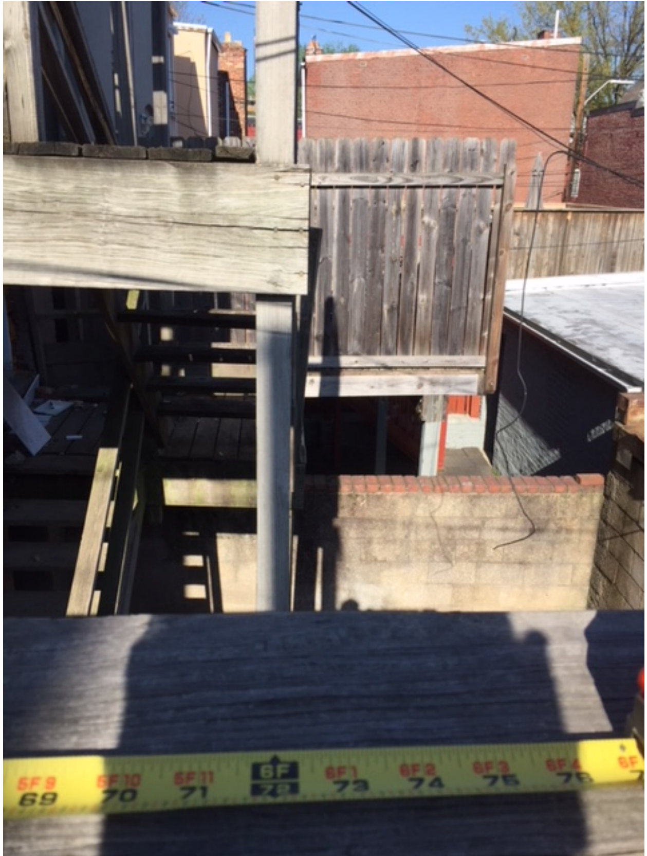
2. Depth of rear stairs from rear façade (May 2, 2018)
