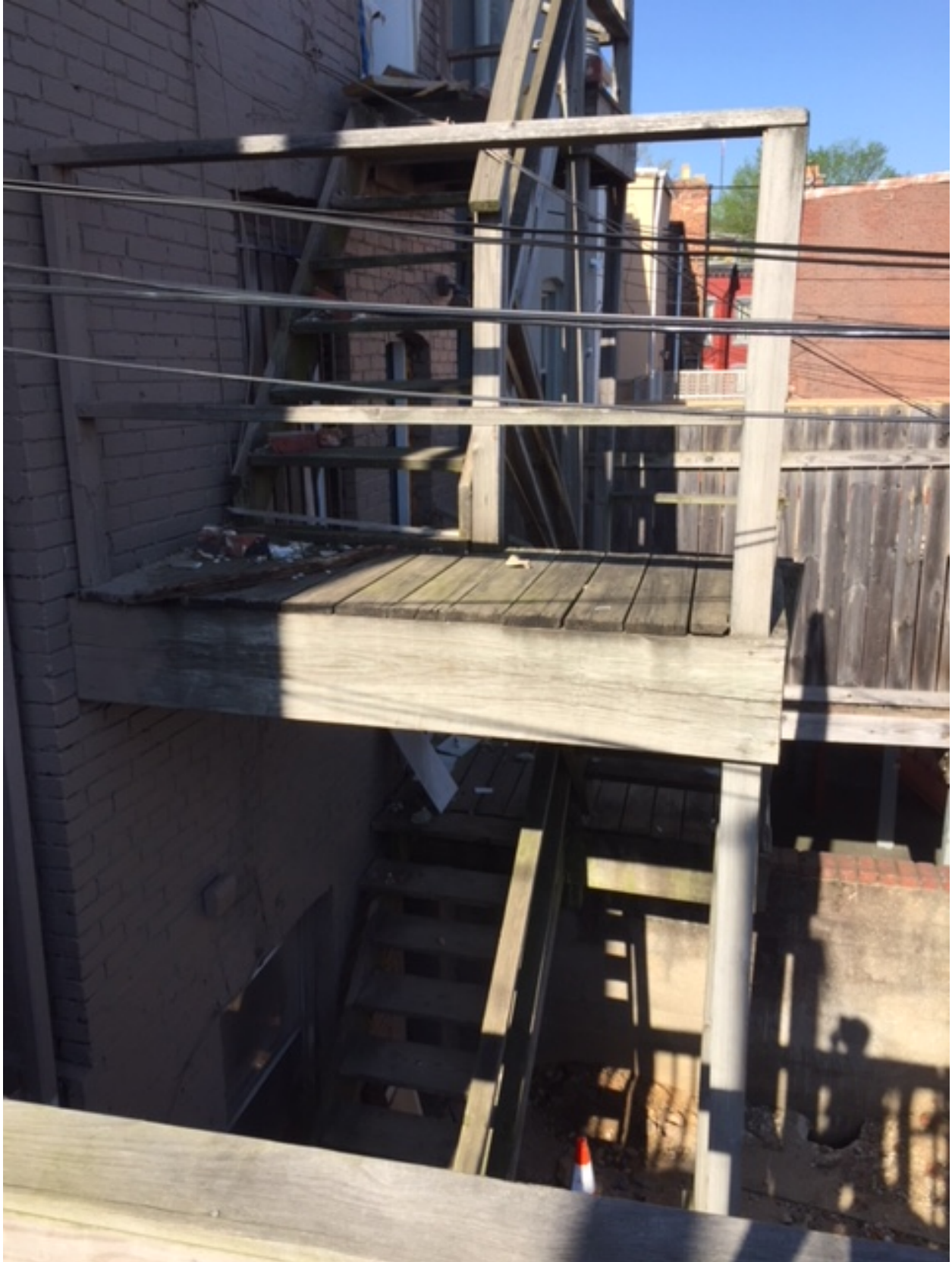
1. Rear exterior stairs (May 2, 2018)
