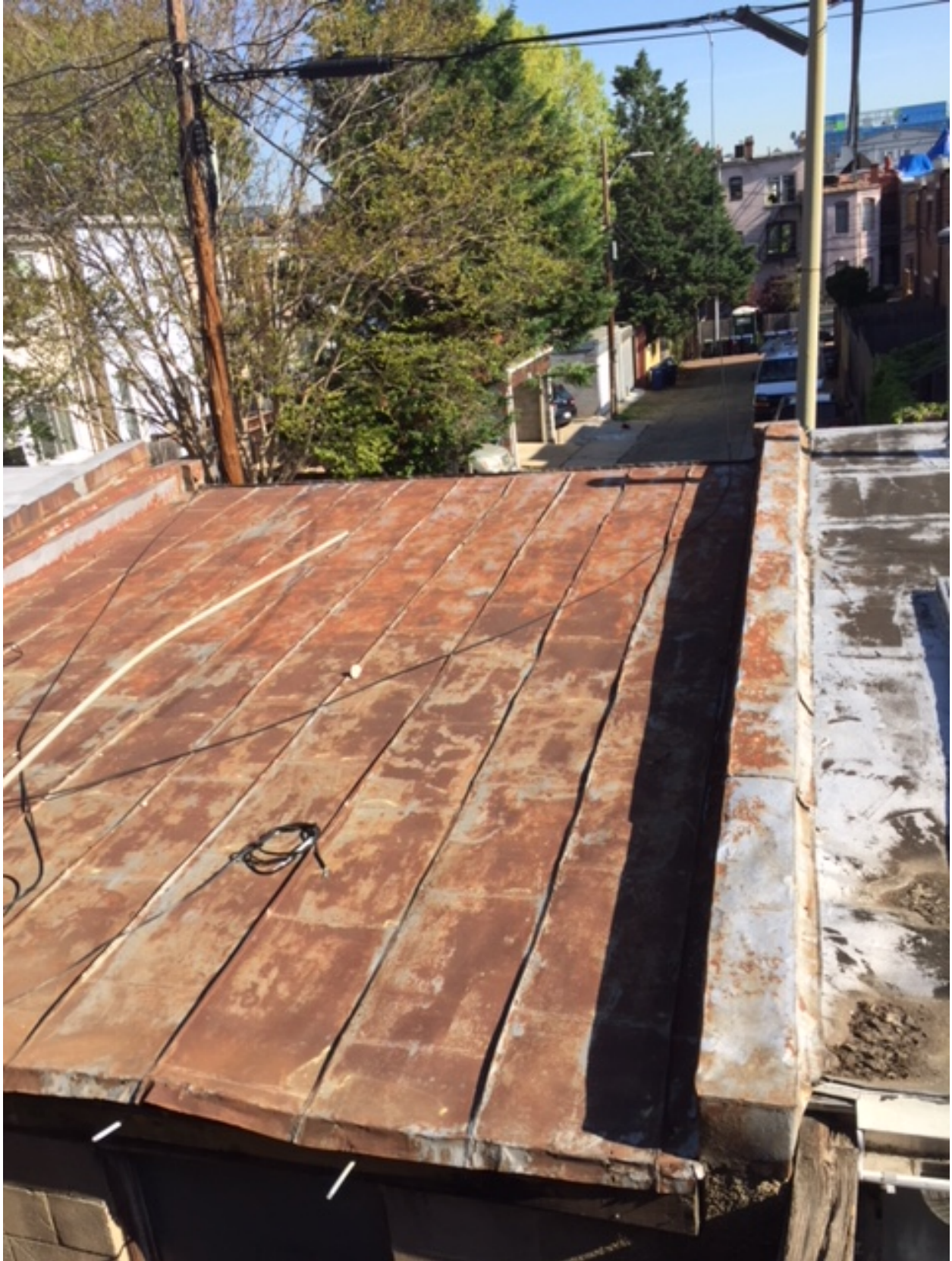
4. 310 E St. NE garage (May 2, 2018)
