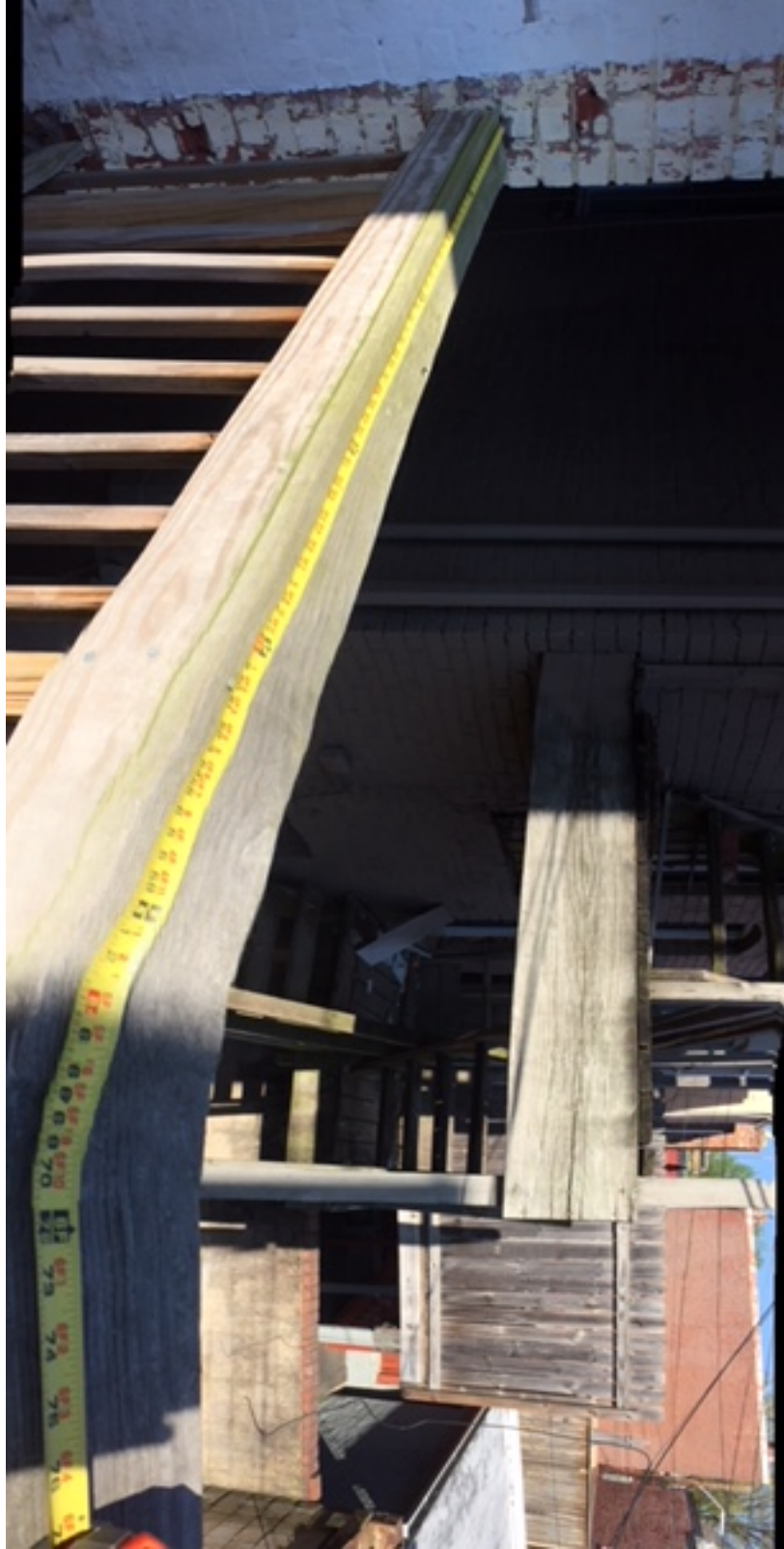
3. Panoramic view of rear stairs measurement (May 2, 2018)
